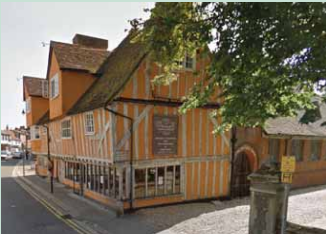
Figure 2.8: Historic building on St Andrew Street
