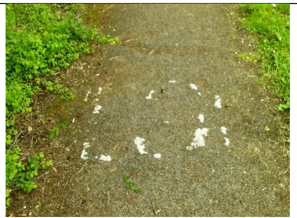
Image 6: Very worn road marking on cycle path to Hertingfordbury.
