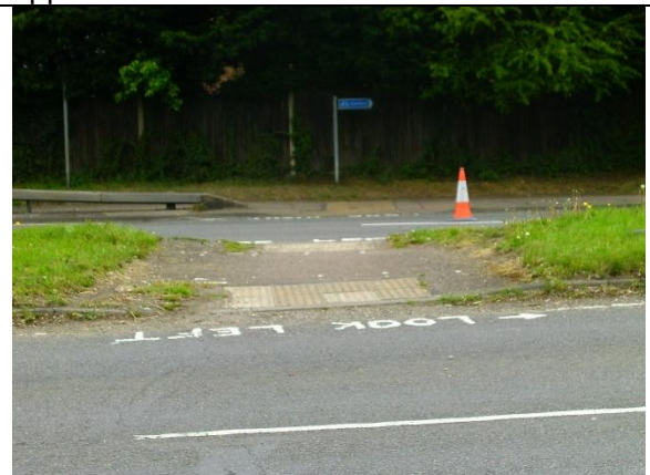
Image 4: Uncontrolled pedestrian/ cycle crossing on A414 to east of Thieves Lane roundabout
